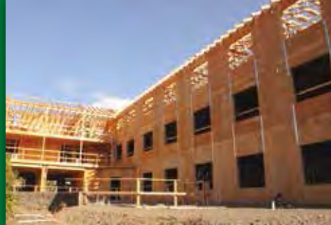
WALL PANELS & IKAIKA EWP @ HOLIDAY INN, KONA
