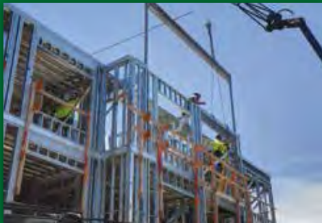
STEEL FRAMING @ KA MALANAI, KAILUA
