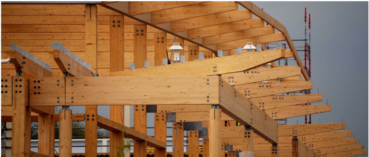
Figure 2. Gluelam usage in load-bearing structures (Timberfreak 2013).
