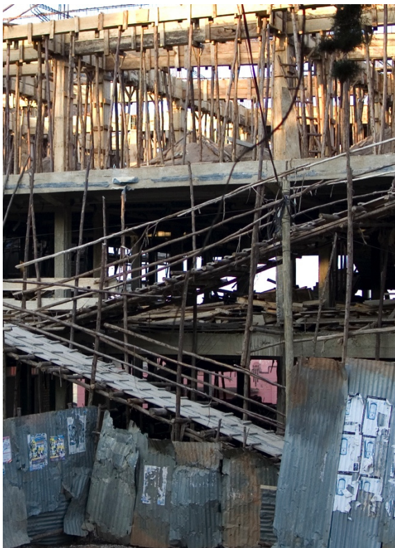
Figure 4.8. Eucalyptus poles used for scaffolding and shoring.
