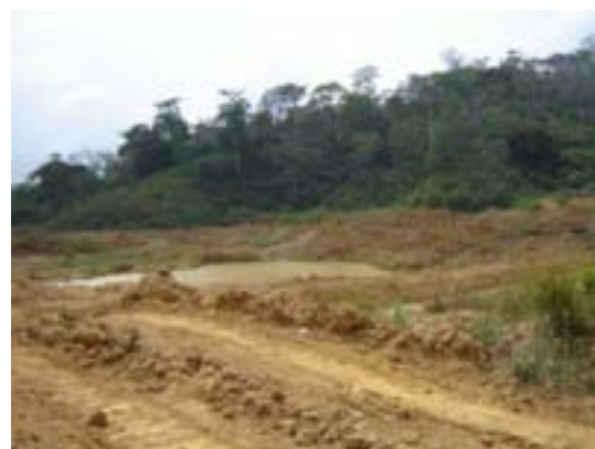
Plate 1. Abandoned licensed surface gold mine at the fringe of Atewa RFR near Kibi
