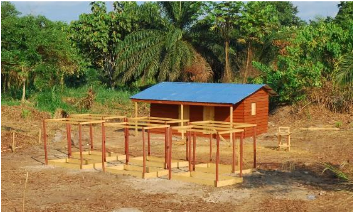
Figure 2. Realization of a nursery and a double hut by ten villagers after the artisanal sawing of two half logs. Makokou, June 2011.
