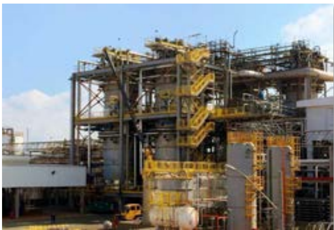
Solazyme Bunge renewable algal oil facility, courtesy of Solazyme.
